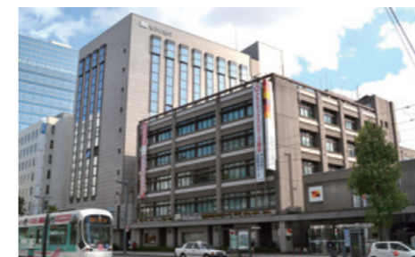
Head office of Momiji Bank, Ltd.
